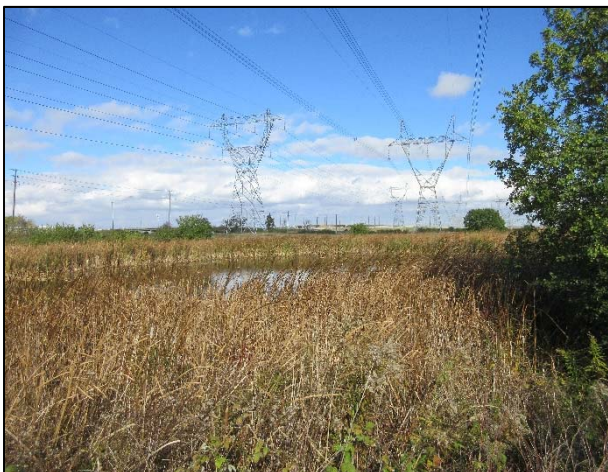
View looking south at MAM/MAS2a with CUT1a to the west.
